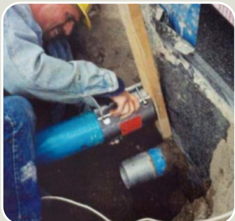
▲ U.S.: sewerage repair work
