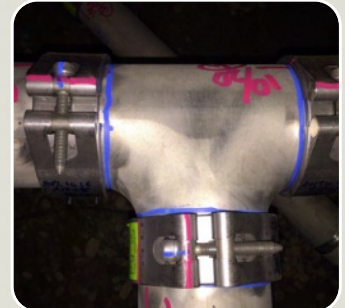
▲ Japan : "T" Repair
