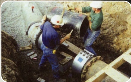
▲ Repair work for pipes replaced underground
