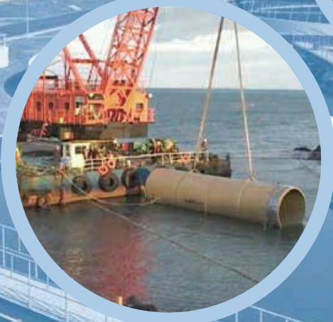
Installation of ocean bed blocks
